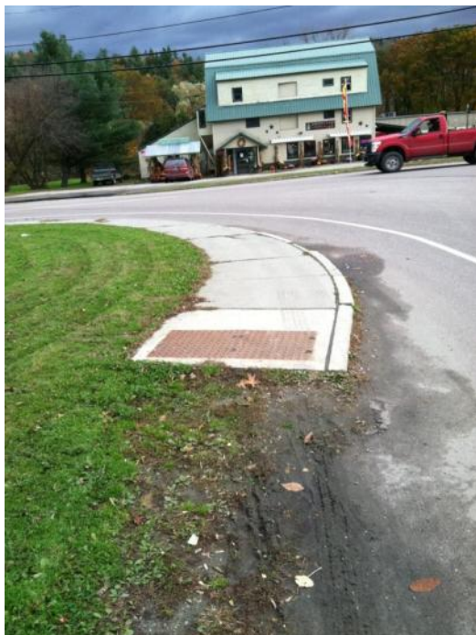
Figure 12: End of sidewalk on northwest corner of US 2- VT 100 (note tire tracks on sidewalk and in mud)
