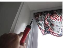
Even newer windows leak at meeting rails and jamb liners. Removable storm panels can be installed in the winter to seal the leaks.
