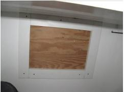
The two photos above show two obvious leaks through the attic plane. On the right, the under insulated attic hatch is also not weather stripped. On the left, the sheetrock edge disappears unsealed behind a beam. It is apparent that air moves through the resulting hidden gap.
