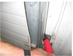
The garage doors have adjustable rollers that can be used to pull the door tighter to the weather stripping or if needed the weather stripping can be installed to meet the doors. In this case it appears that the installation is adequate until there is wind pressure on the doors. With wind on the doors, there is a gap of <sup>1</sup>/<sub>4</sub> inch or more. Weather stripping should be inspected annually and repaired or replaced as needed.
