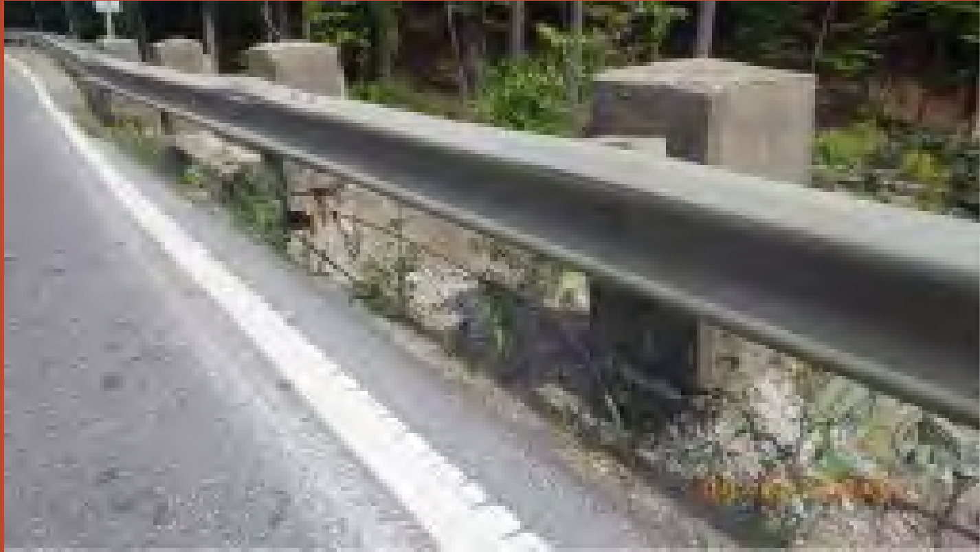
Existing Bridge Railing Posts
