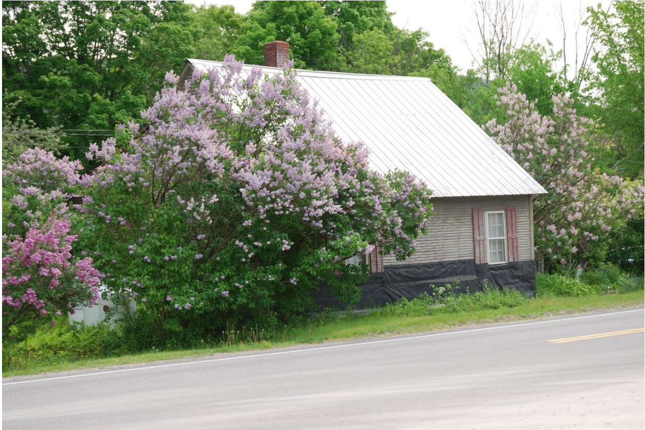
Photo 32. View of Structure 12 at 452 Route 2, looking east.
