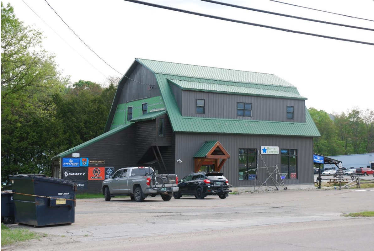
Photo 8. View of Resource 2 at 23 Commercial Drive, looking east.
