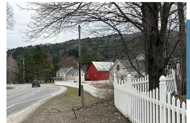
Fence to be removed and reset; telephone pole to be relocated. Tree roots may be impacted.
