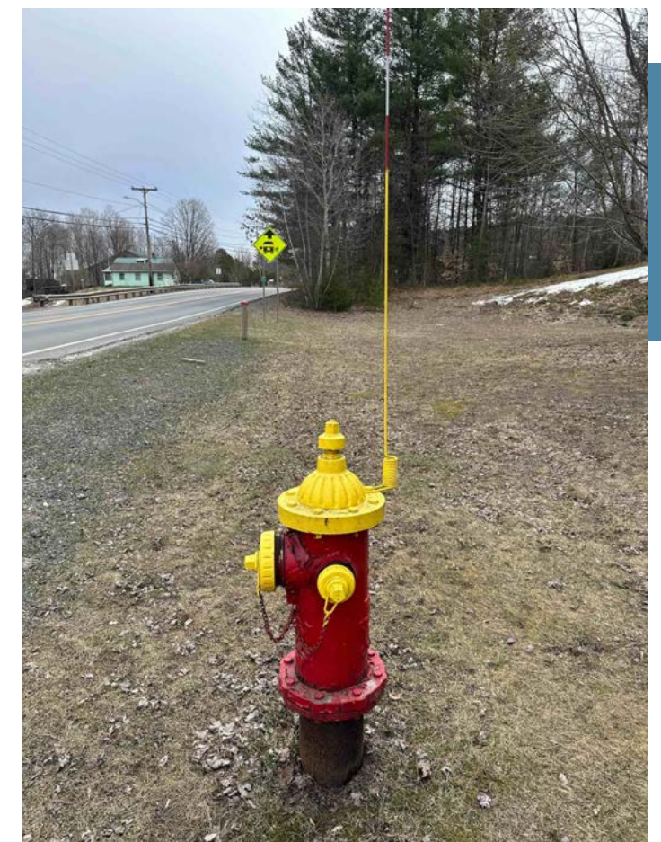
This hydrant may need to be moved in Concept 2.
