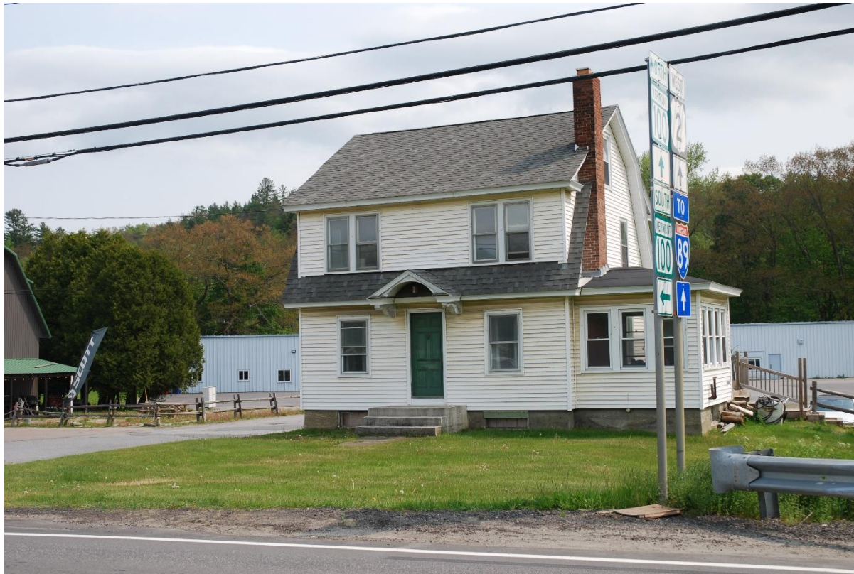
Photo 11. View of Resource 3 at 16 Commercial Drive, looking north-northeast.
