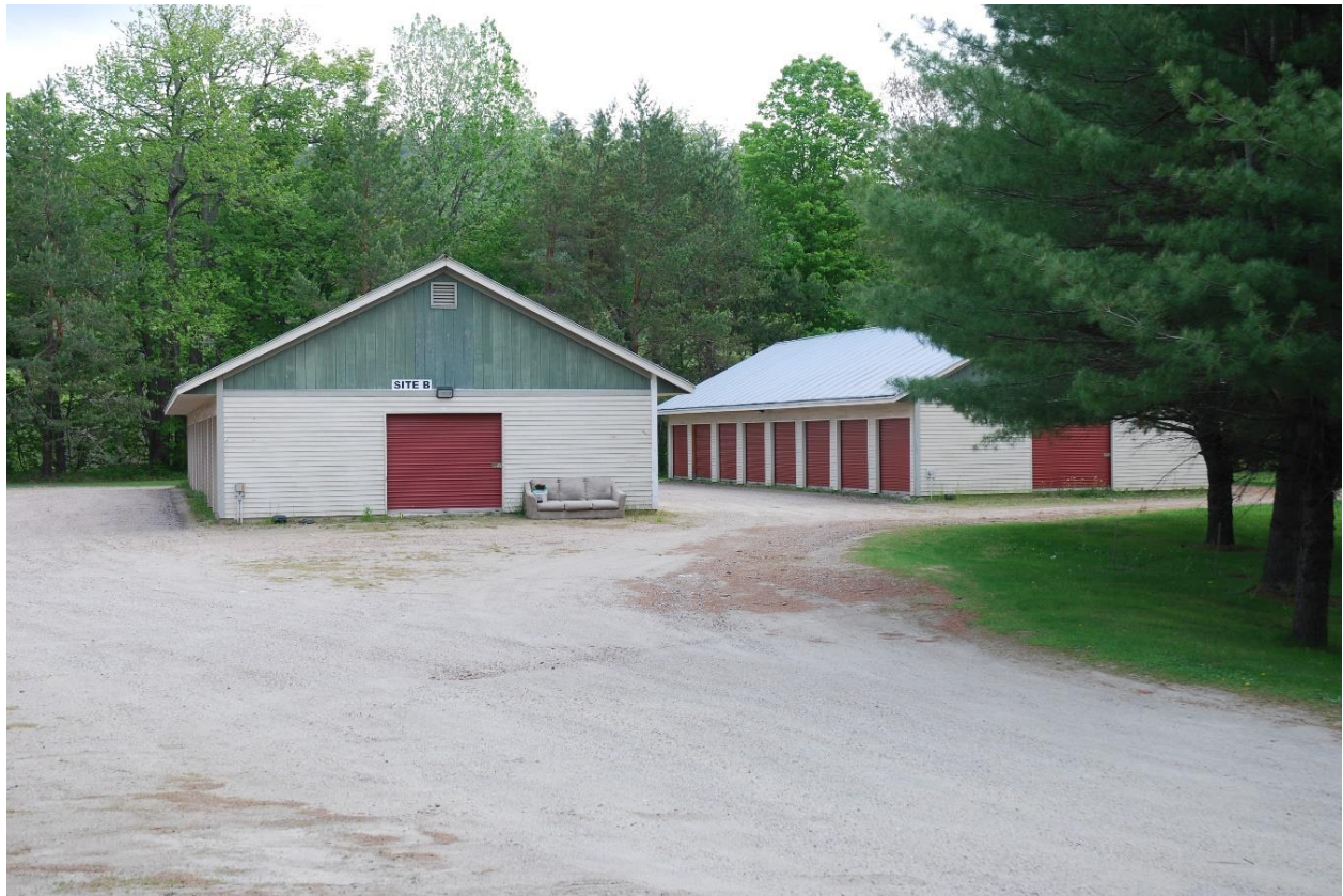
Photo 15. View of structures associated with Resource 5 at 251 Route 2, looking east-northeast.
