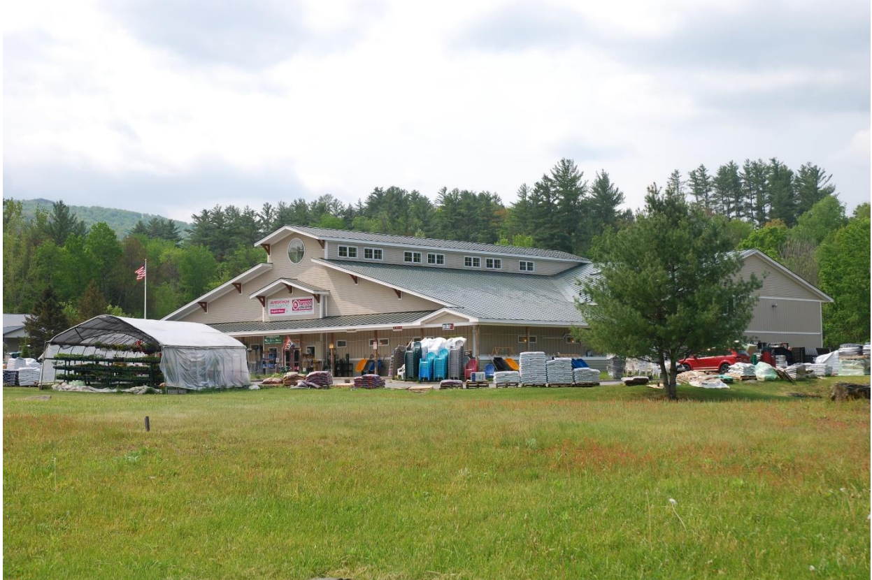
Photo 47. View of Resource 20 at Mason Drive, looking south-southwest.
