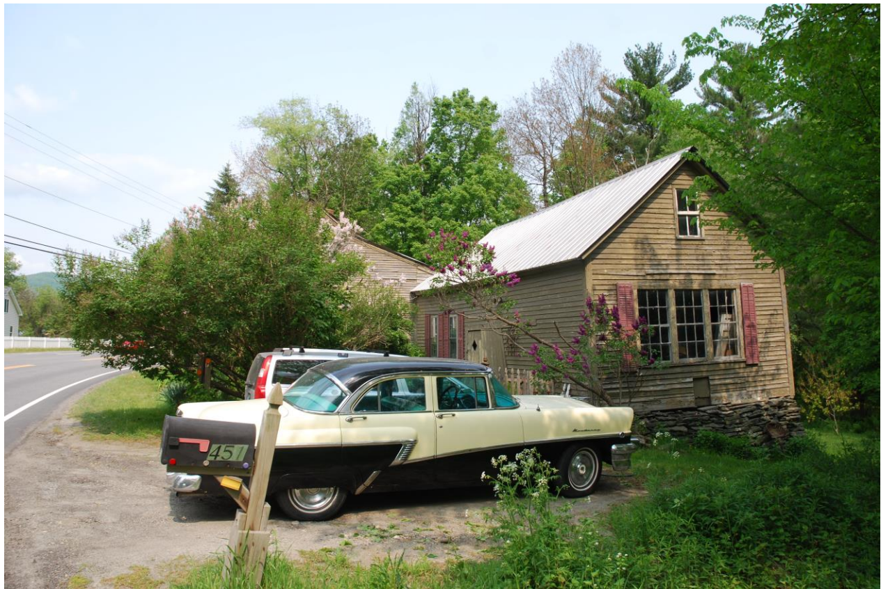
Photo 31. View of Structure 12 at 452 Route 2, looking west-northwest.
