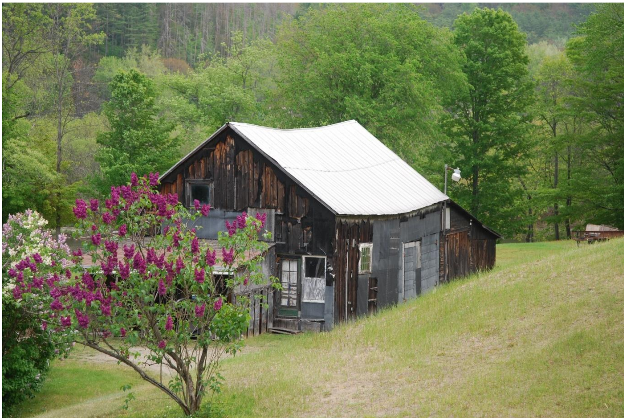
Photo 20. View of structure associated with Resource 7 at 313 Route 2, looking east.
