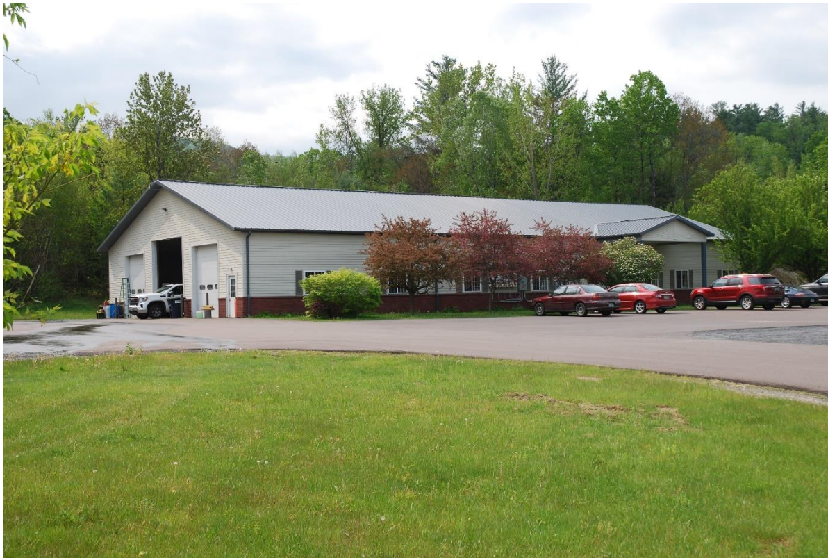
Photo 44. View of Resource 19 at Mason Drive, looking south-southwest.
