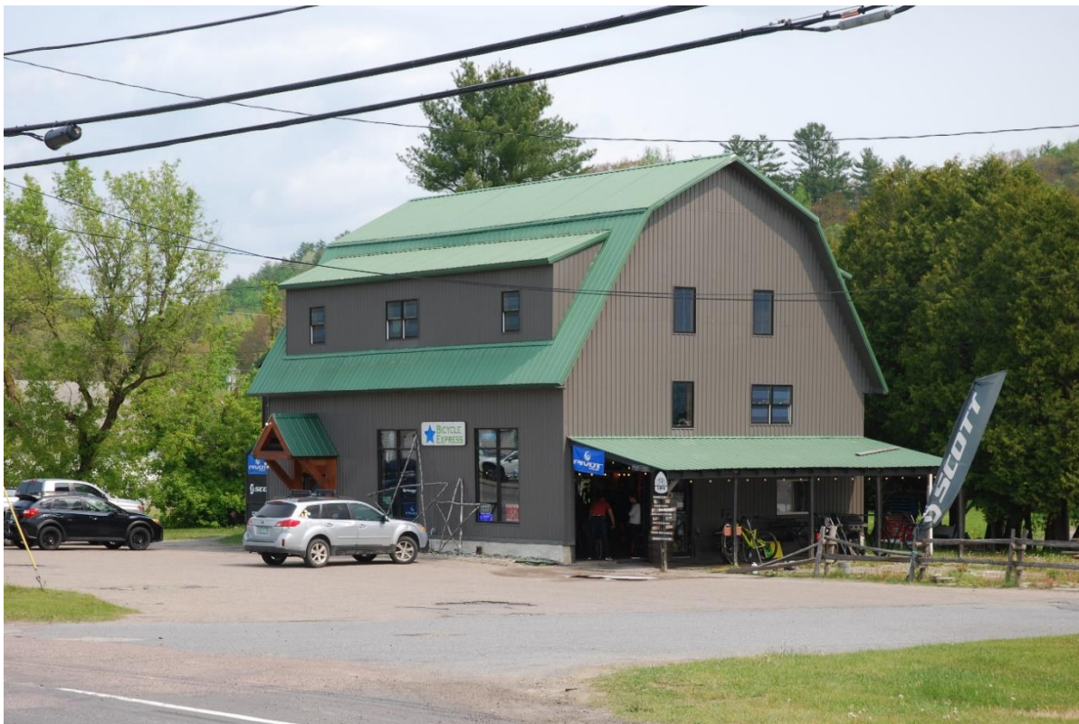
Photo 9. View of Resource 2 at 23 Commercial Drive, looking north.
