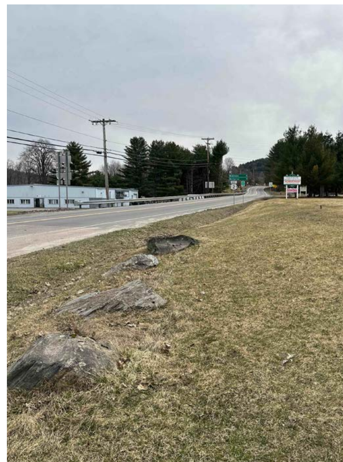
This swale in front of Aubuchon Hardware is preserved in Concept 2. However, the path itself may cross property lines to make room.
