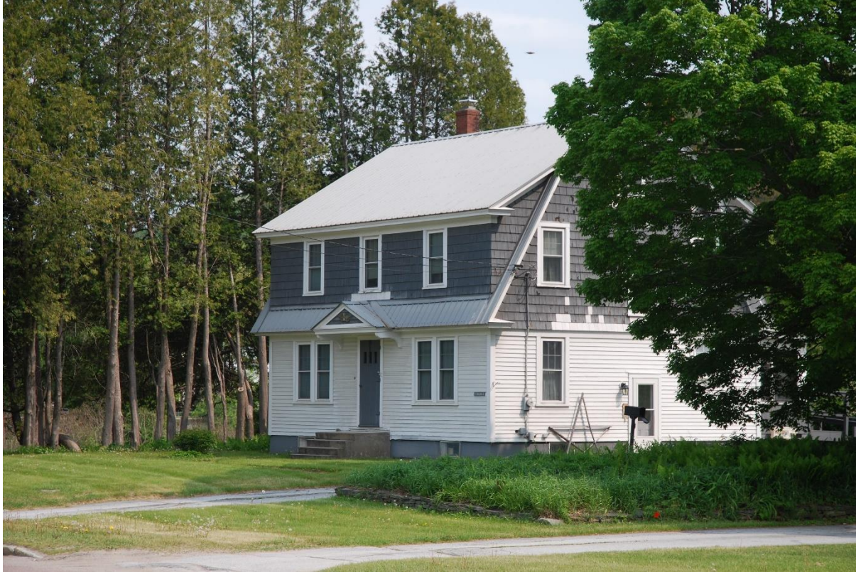
Photo 5. View of Resource 1 at 71 Route 2, looking north.
