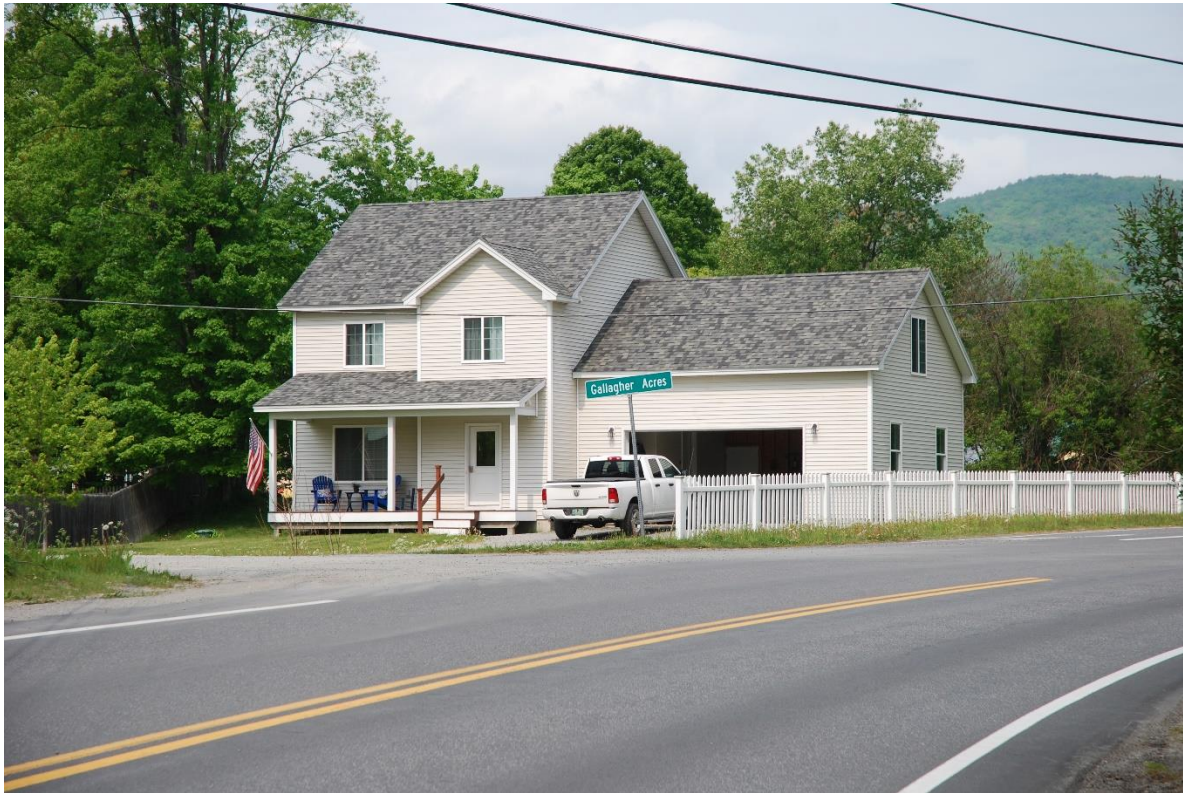
Photo 37. View of Resource 15 at 18 Gallagher Acres, looking west.
