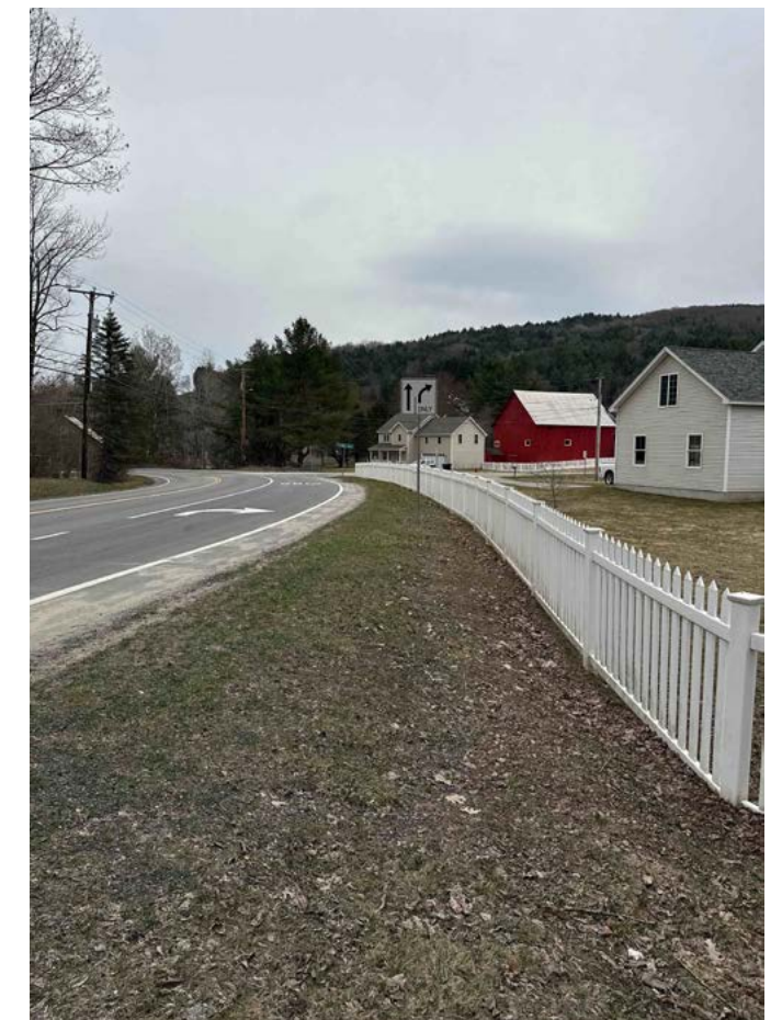
This fence will have to be removed and reset during construction.
