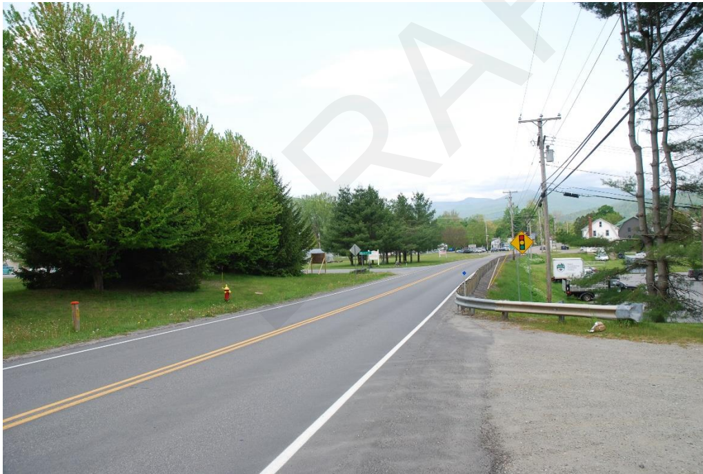
Photo 3. View along US Route 2. Note the sharp slope down on the east shoulder of the road and fire hydrant on the west side indicating buried utilities in that area. View facing northwest.
