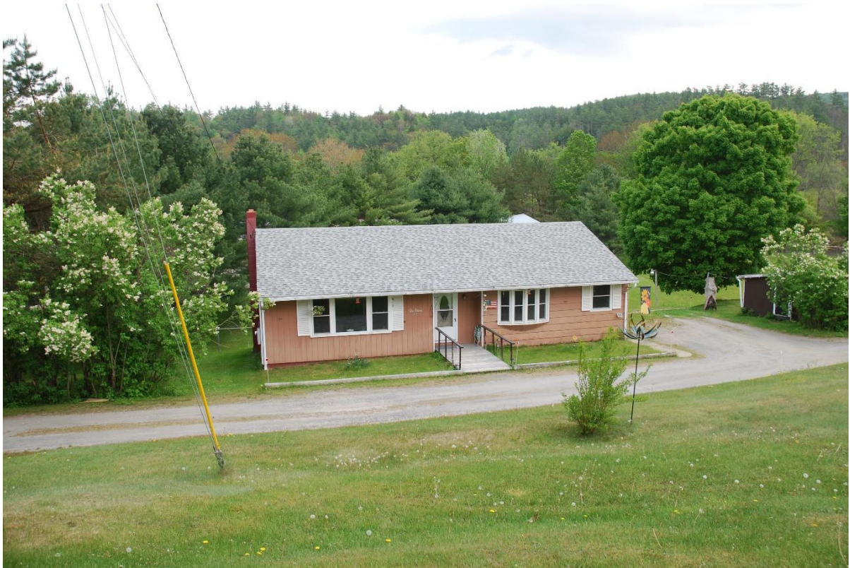
Photo 17. View of Resource 6 at 253 Route 2, looking north-northeast.
