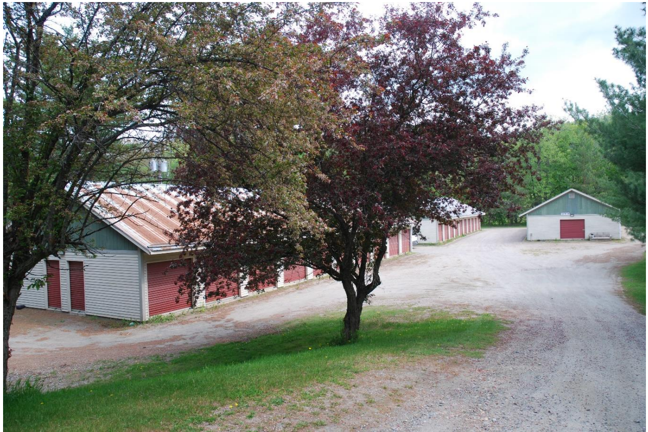
Photo 14. View of structures associated with Resource 5 at 251 Route 2, looking northeast.
