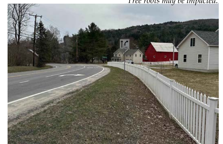
Fence to be removed and reset.
