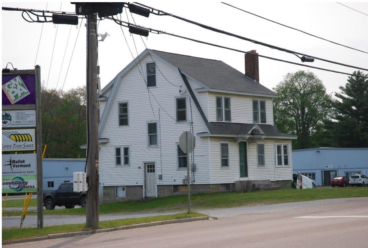
Photo 10. View of Resource 3 at 16 Commercial Drive, looking southeast.
