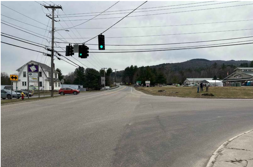
A view southeast into the project area showing the intersection of US-2 and VT-100. Note the existing sidewalk (bottom right) and its lack of crossing connections through the intersection.
