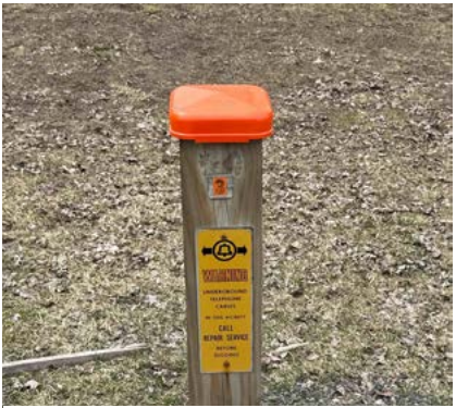
A marker indicating the presence of buried telephone lines nearby
