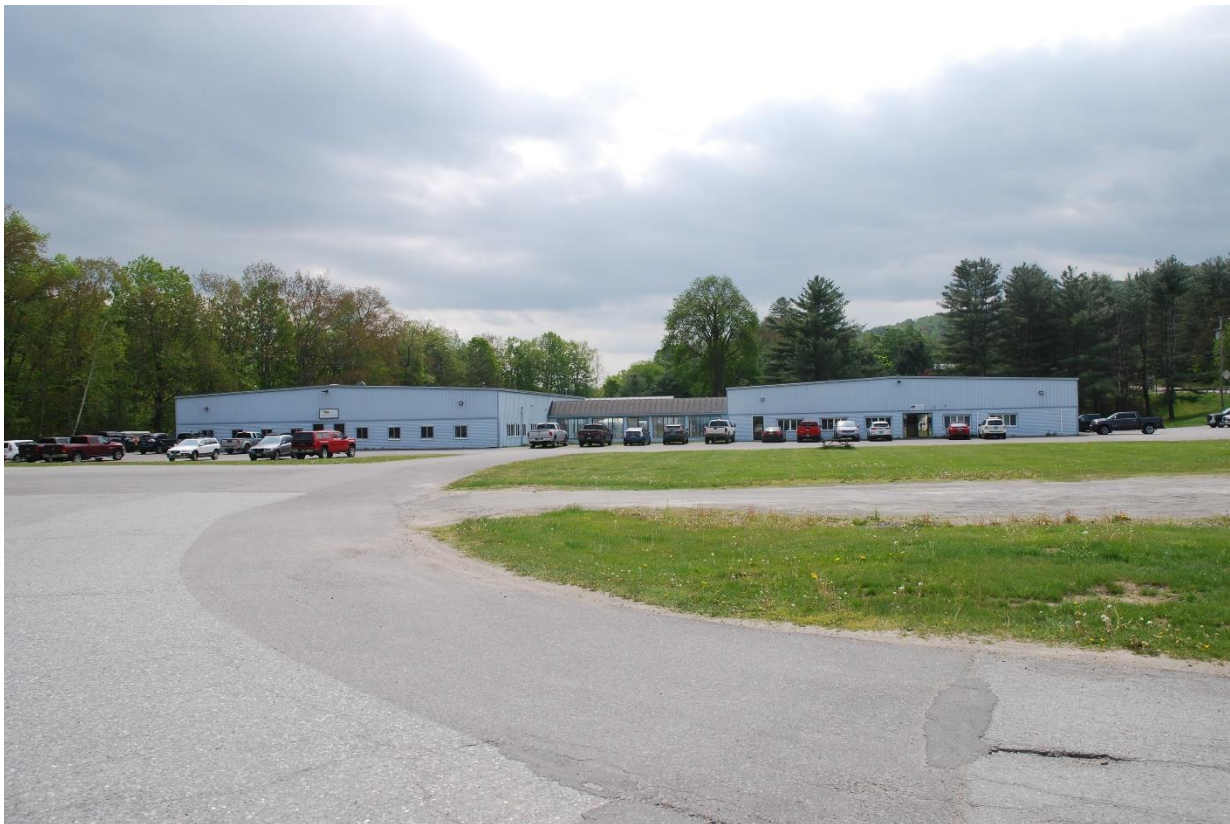
Photo 13. View of Resource 4 at 80 Commercial Drive, looking southeast.
