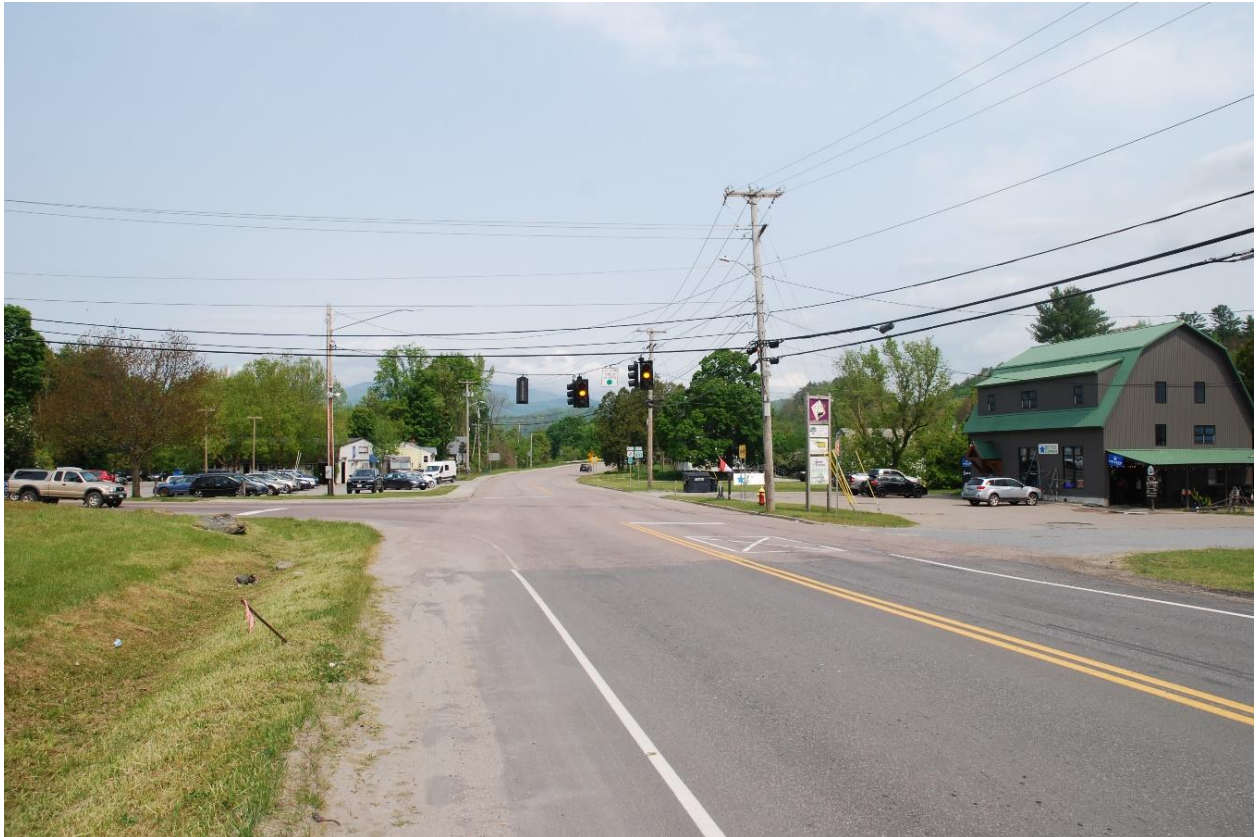
Photo 1. View of Route 100 and Route 2 intersection, looking northwest.
