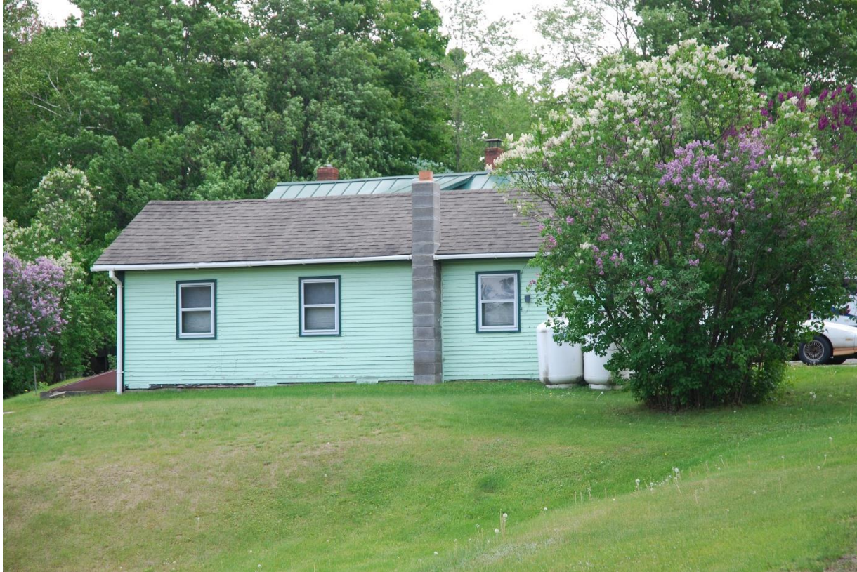
Photo 19. View of Resource 7 at 313 Route 2, looking east-southeast.
