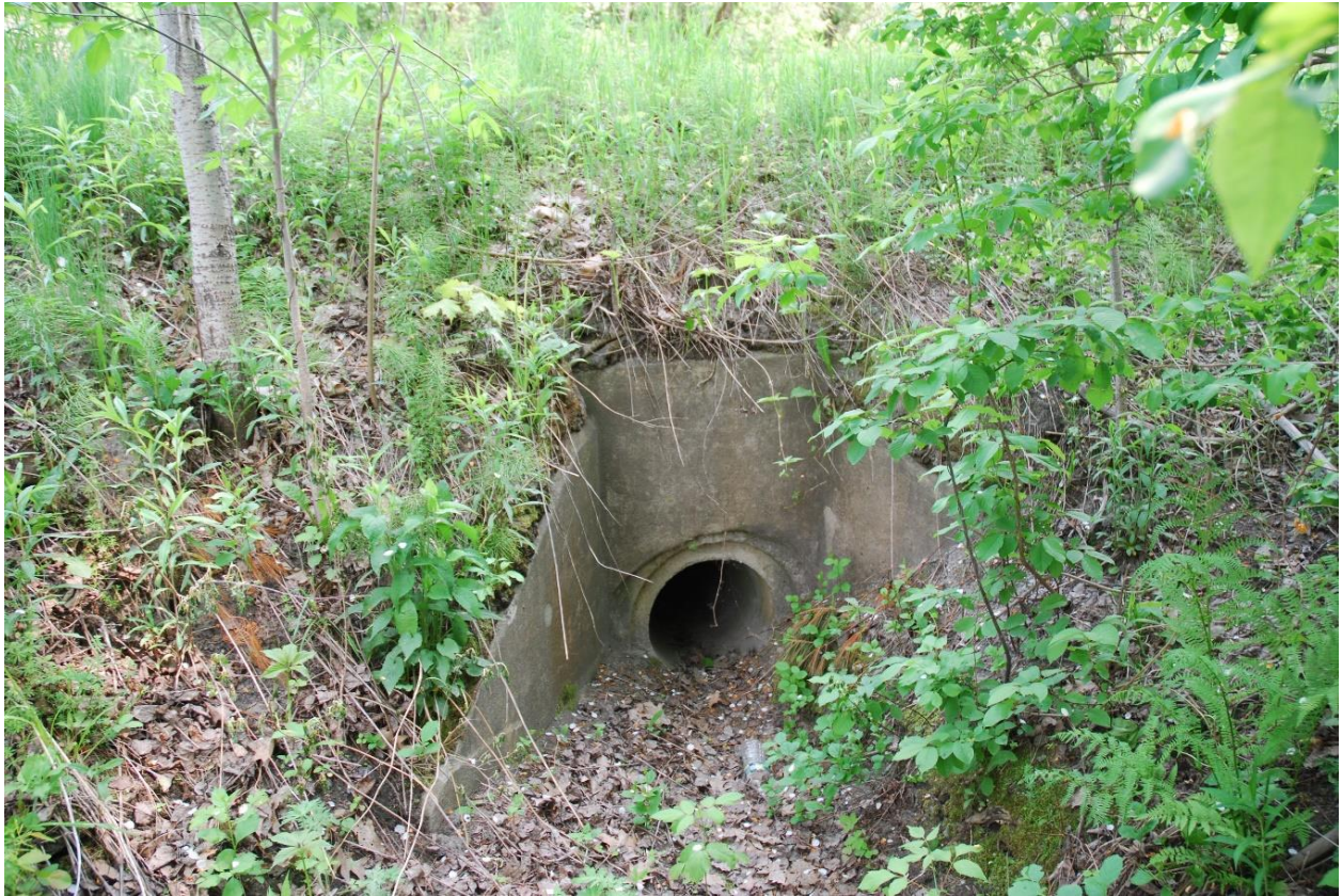
Photo 33. View of Resource 13, looking north-northeast.
