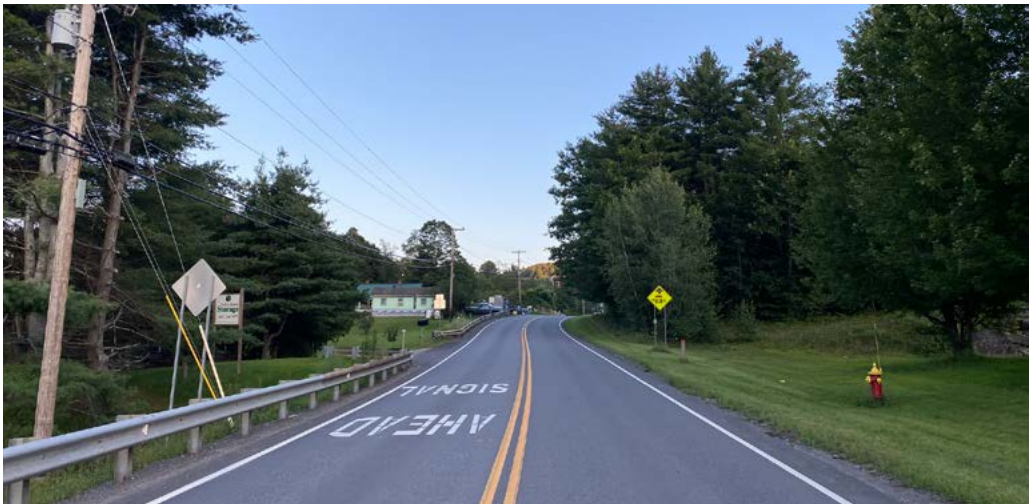
Eastward view of US-2 in the project area. The straight road provides good sight-lines for drivers.
