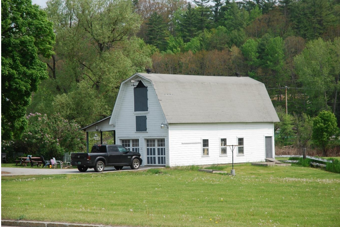
Photo 7. View of structure associated with Resource 1 at 71 Route 2, looking north-northeast.
