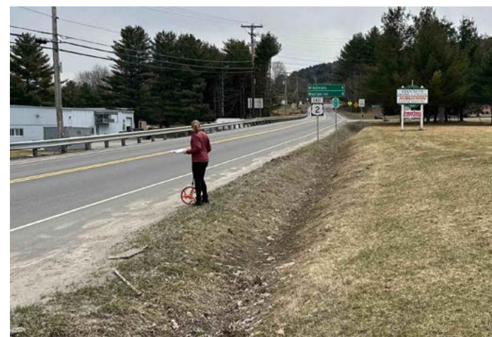
Existing swale to remain in front of Aubuchon Hardware.
