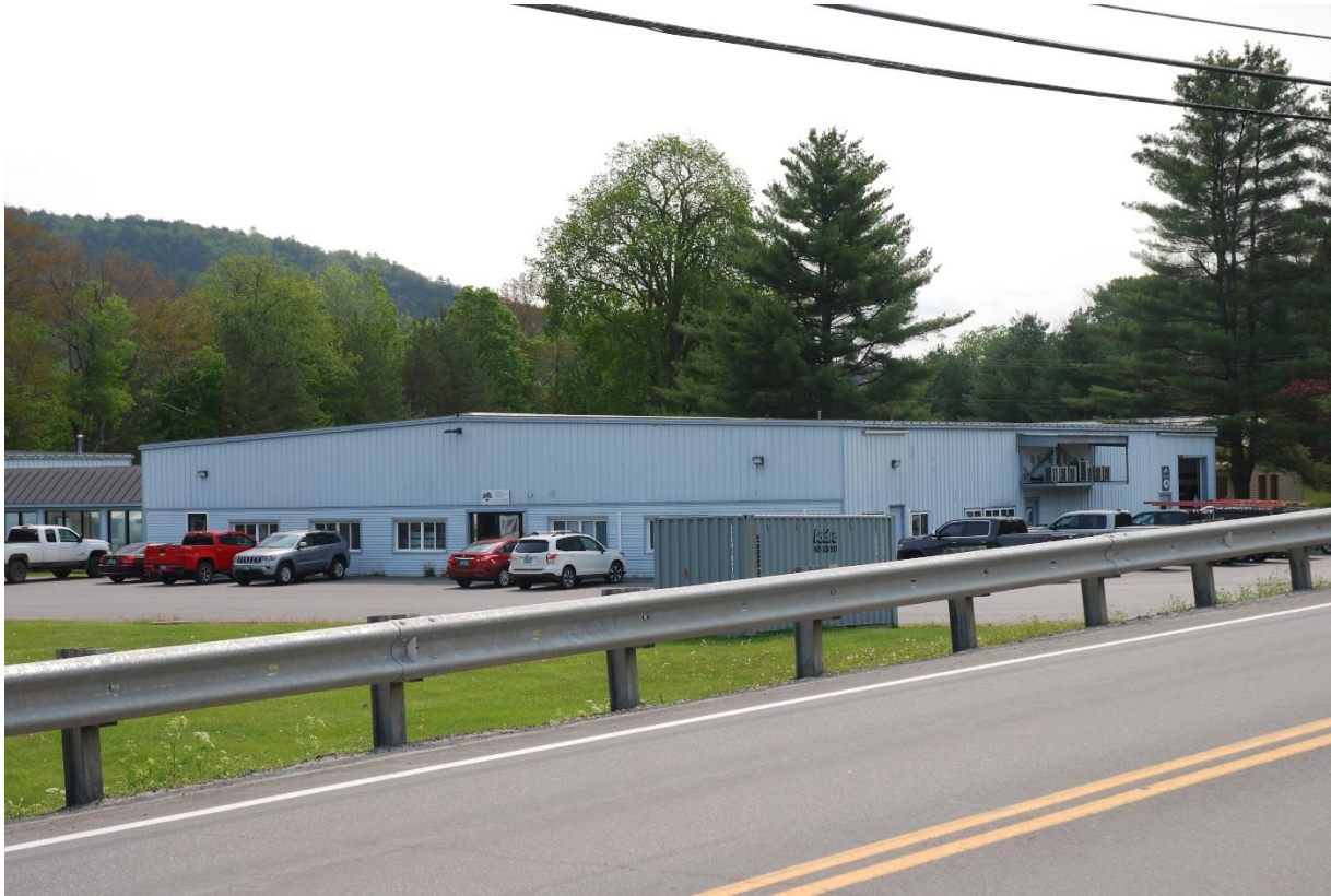
Photo 12. View of Resource 4 at 80 Commercial Drive, looking east.
