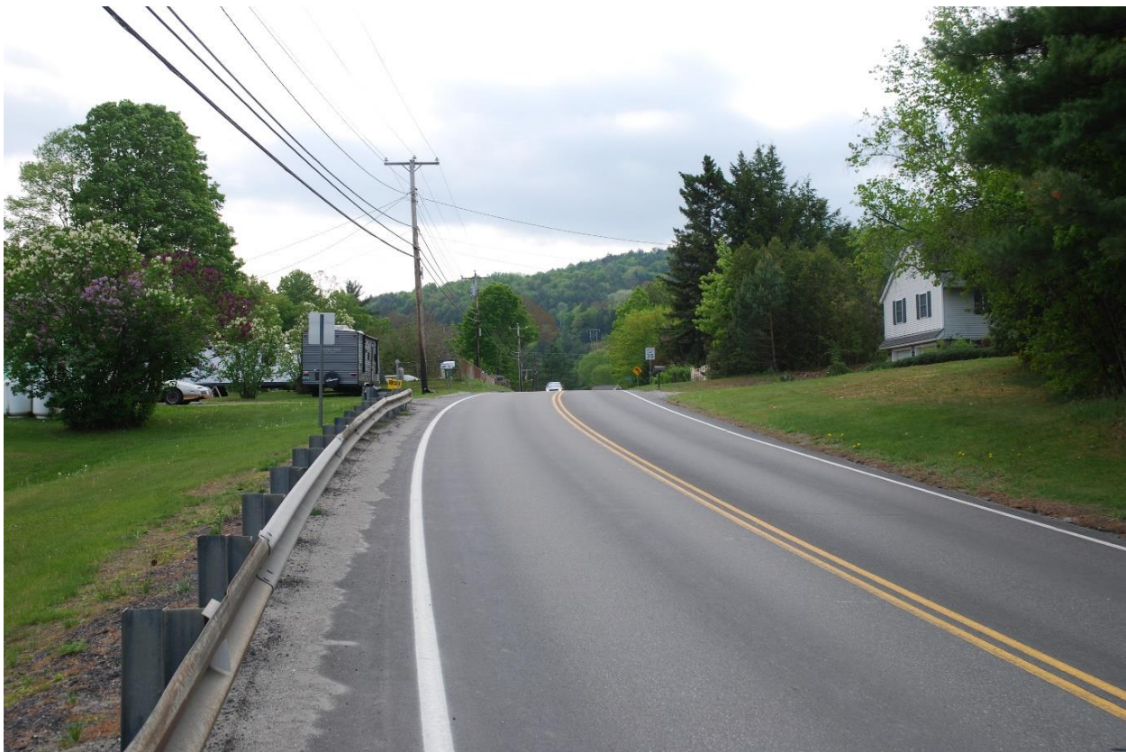
Photo 3. View looking southeast from Resource 5.
