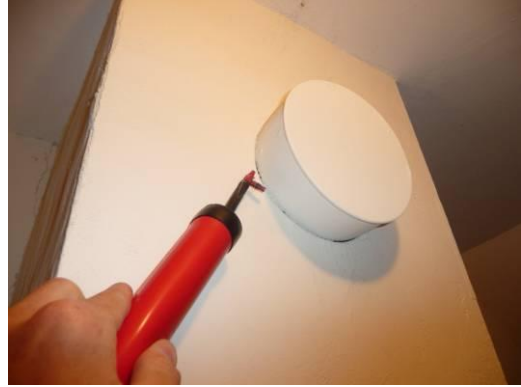
The open chimney thimble in the basement is a major source of air leakage. This should be plugged and air sealed. The thimble on the second floor is plugged, but it needs to be air sealed.
