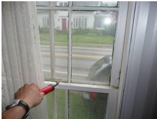
Windows are a source of air leakage, however, addressing the heat loss in the attic and basement areas is a much higher priority. Windows should be adjusted so they close tight in the winter. The exterior storm windows do help reduce heat loss. The interior window trim can be removed and the shim space air sealed with low expansion foam sealant. In the future, the windows can be replaced.
