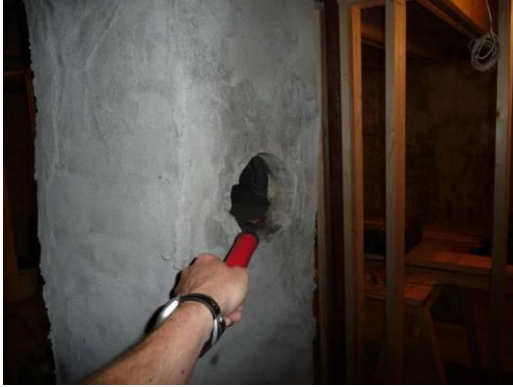
The open chimney thimble in the basement is a major source of air leakage. This should be plugged and air sealed. The thimble on the second floor is plugged, but it needs to be air sealed.
