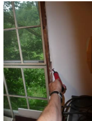
Windows are a source of air leakage, however, addressing the heat loss in the attic and basement areas is a much higher priority. Windows should be adjusted so they close tight in the winter. The exterior storm windows do help reduce heat loss. The interior window trim can be removed and the shim space air sealed with low expansion foam sealant. In the future, the windows can be replaced.
