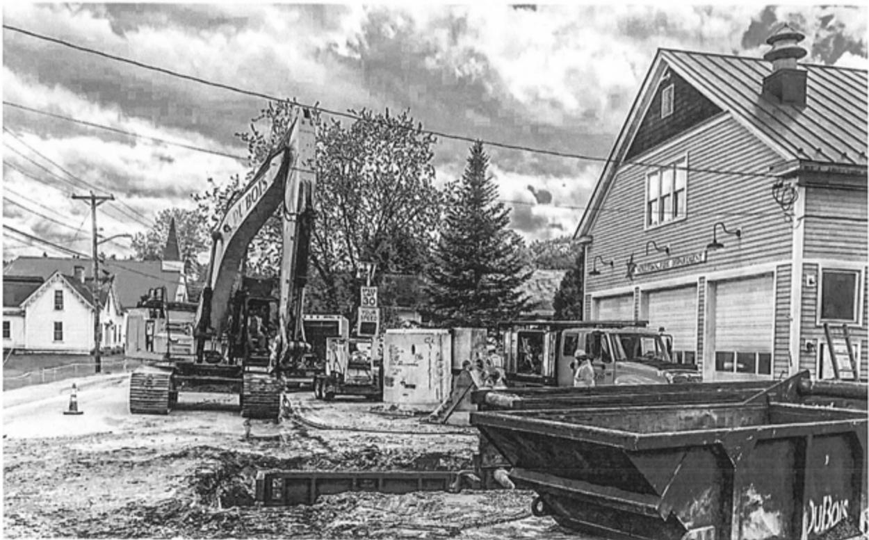
Catch Basin work at the Fire Station Summer 2020 – preparation of the East side of the sidewalk construction
